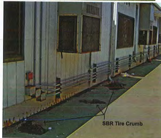
Intake ducts and drifts of SBR Tire Crumb
