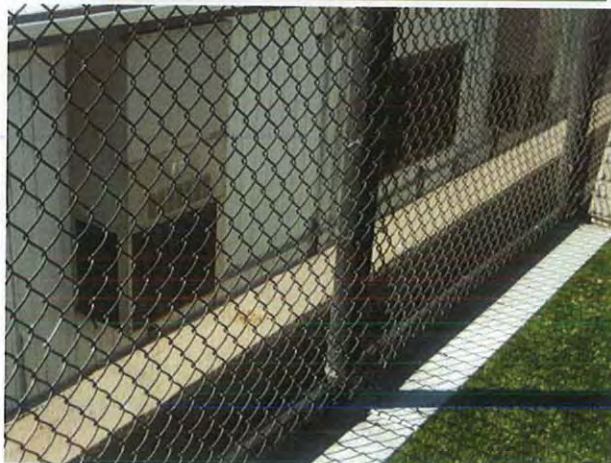
Classroom intake ducts
